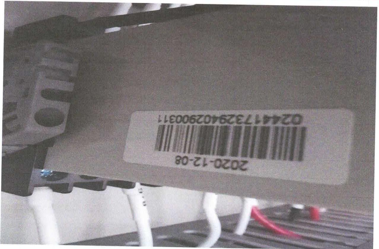
34 RELAY, TIME DELAY, MODEL JSZ3, AC 50HZ/60HZ, 24 VDC
